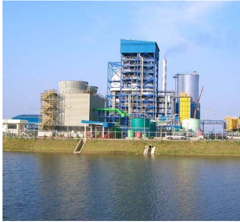
A.T. Biopower 20 MW Rice Husk-Fuelled Power Plant Thailand
